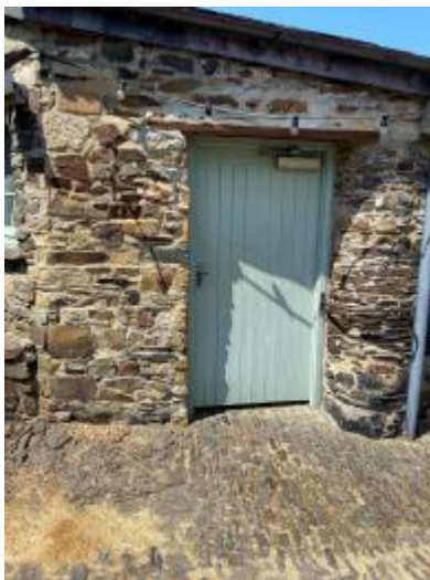
Door to Courtyard Toilet
